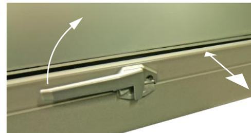
For awning windows without chainwinders (& all casements), **latches** are fitted. Rotating the handle unlatches the sash from the closed position, allowing the window to be opened. Reverse actions to close
